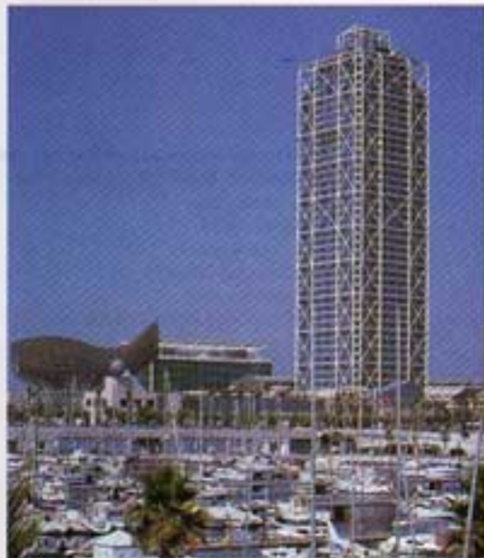
Above and below: The Hotel Arts tower, designed by SOM's Bruce Graham, is encased by an exposed steel exoskeleton. Frank Gehry's magnificent fish sculpture of woven, anodized aluminum strips crowns his retail center, adjacent to the hotel's terraces and gardens.
